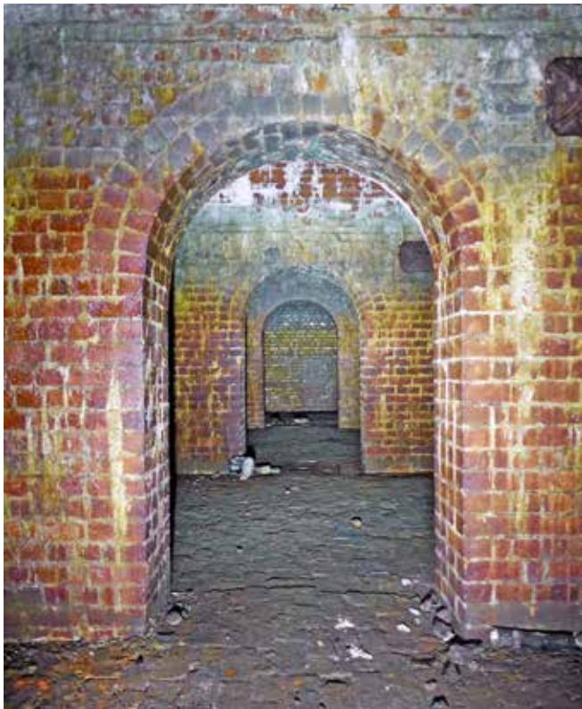
One set of inter-connecting archways, looking across all four chambers
